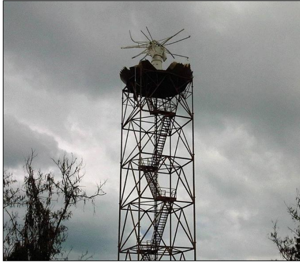
Figure 1-11. Kadena Air Base Doppler weather radar, damaged by passage of STY 04W.
